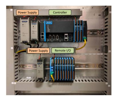
Figure 3.2 AMAX-5000 installed in control box
